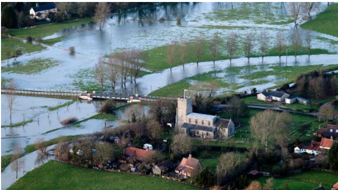
Flood (out of bank): Water has breached the riverbank on one or both sides of the river channel.
