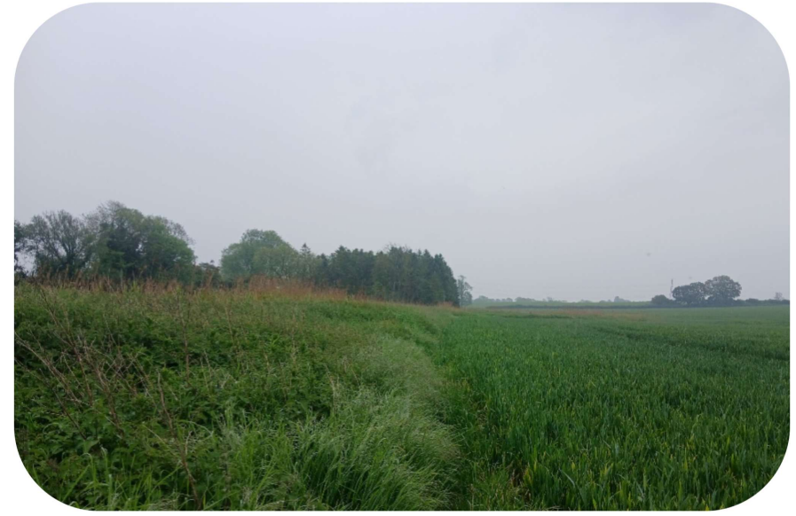
Embankment along this reach of the Pant. The embankment is around 1–2m high compared to the floodplain. The Pant is not visible here due to the embankment and incised channelling, but in places the channel is around 4m deep or more.
